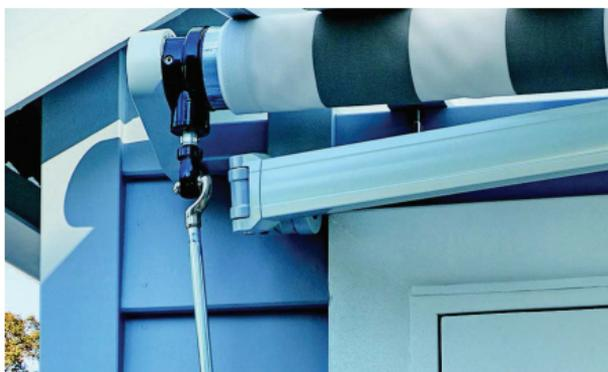
2. Wind handle clockwise and allow awning to extend to the desired projection.
